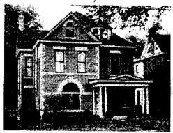
renovation of one of the upstairs apartments. Most visible of all the repairs to this historic house was the reconstruction of the parlor (decorative) window, which had previously been removed from the house and the construction of the front porch. The window reconstruction included extensive masonry repair and the creation of an ornate mullion for the center of this two-part window.
